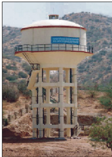
Construction of the over-head pump at Sirohi, Rajasthan, by Dr. Abhishek Singhvi
