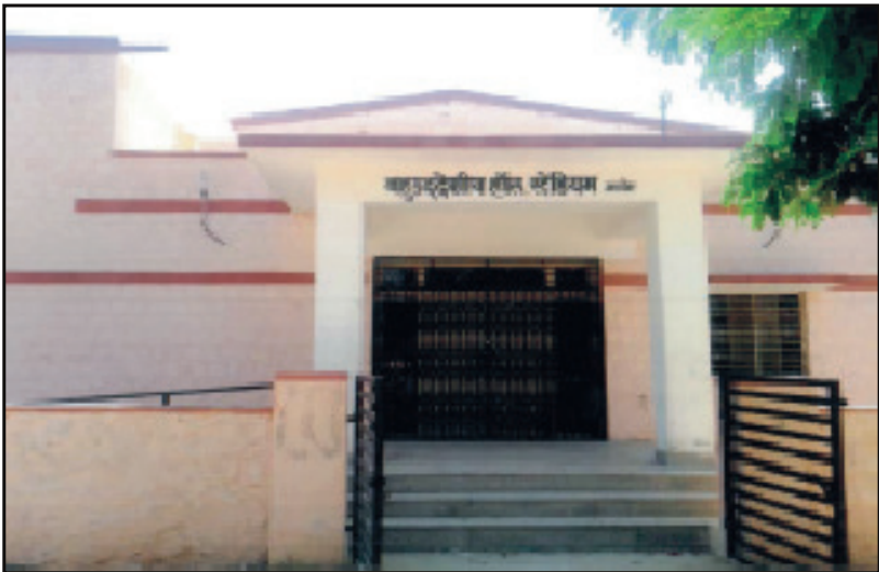
Construction of Auditorium at District Headquarter, Jalore, Rajasthan, by Dr. Abhishek Singhvi
