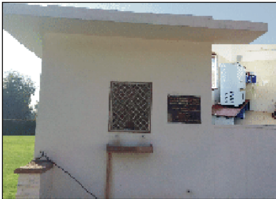
Construction of pyau at Police Commissioner Office, Jodhpur, Rajasthan, by Dr. Abhishek Singhvi
