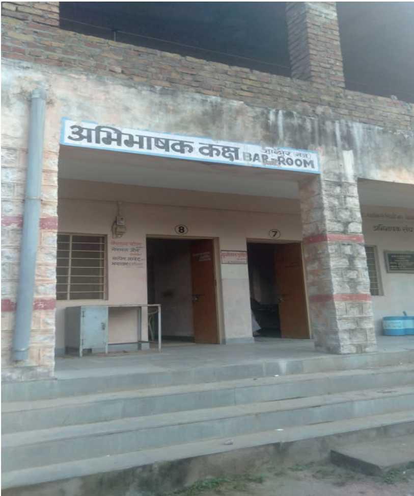
Construction of Bar Room at Jalore, Rajasthan, by Dr. Abhishek Singhvi
